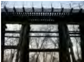
A RELIC FROM RAILROADING'S PAST: Though they pose a maintenance challenge, the Colebrookdale Railroad's bridges provide spectacular examples of early railroad engineering and, as contributing feature's to the line's unique character, should be considered assets.
