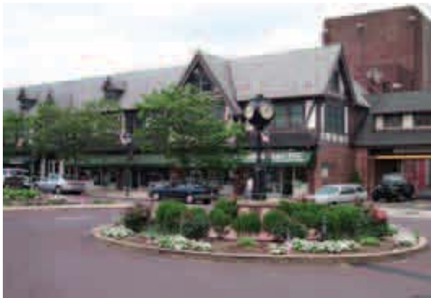
New roundabout, Keswick
