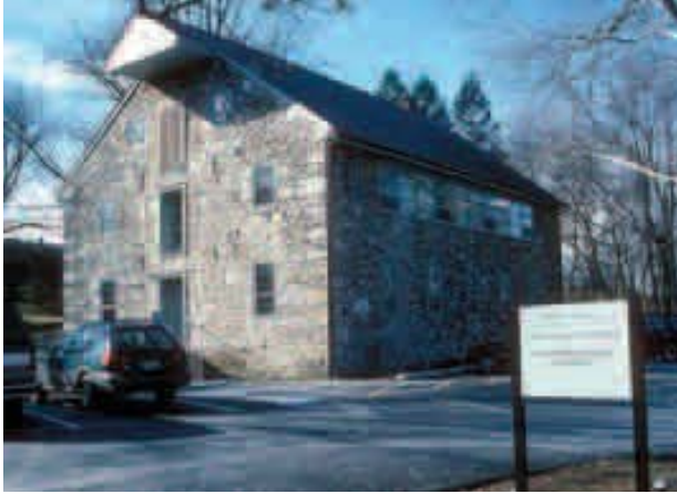
Berks County Conservancy in restored mill building
