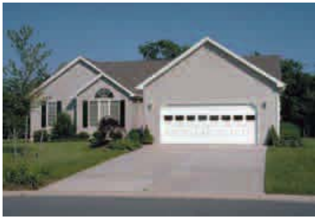
Front yard garage
