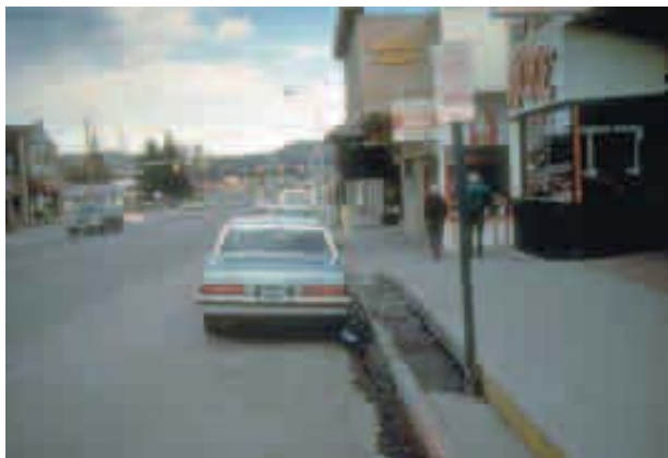
Commercial district with no landscaping
