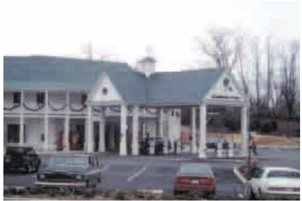
New service station in Virginia has a standing seam metal roof like other nearby buildings.
