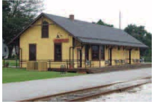
New Freedom train station after rehabilitation
