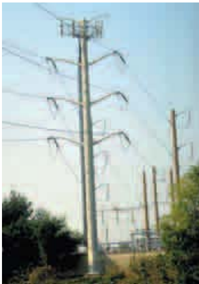
Cell tower on electric lines
