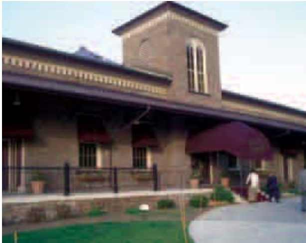
Restored train station, Phoenixville
