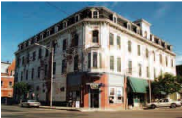
Historic building in Sayre before restoration
