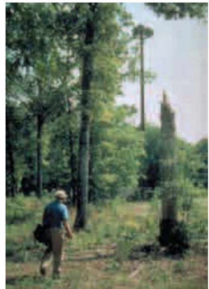
Cell tower disguised as tree
