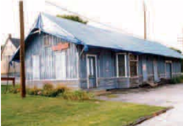
New Freedom train station before rehabilitation
