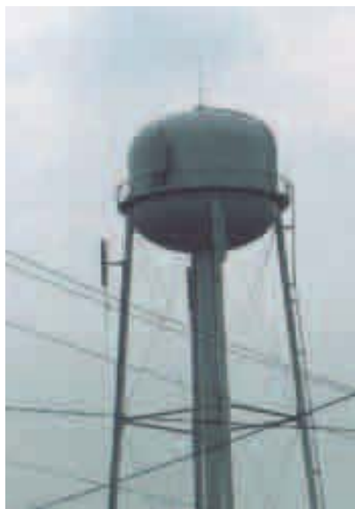
Combined cell/water tower
