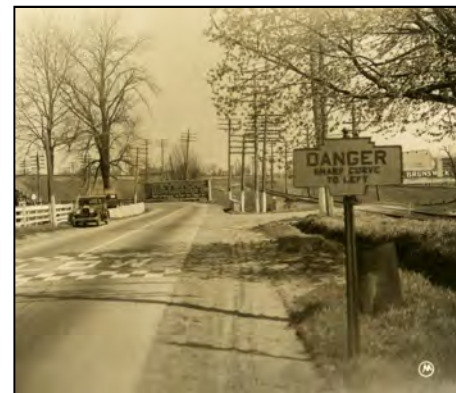
FIGURE 7: ORIGINAL PHOTO OF FRONT-MOUNT “DANGER” SIGN AND POST.
