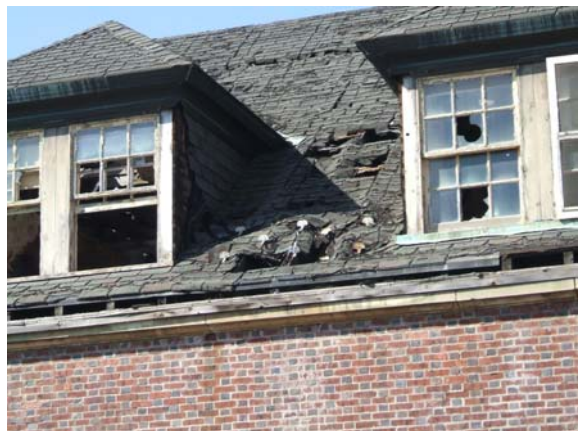
Dietary Building/Franklin Hall Roof
