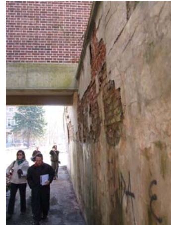
Hospital Retaining Wall
