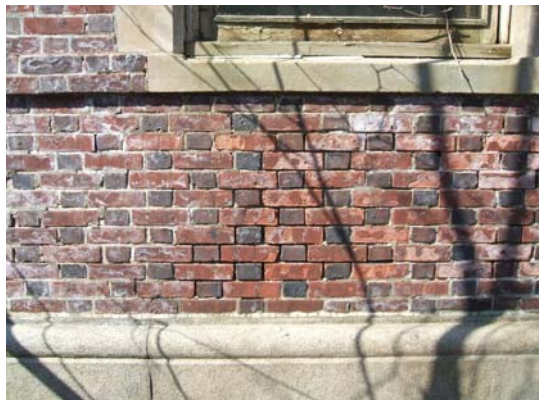
Administration Building Mortar Joints
