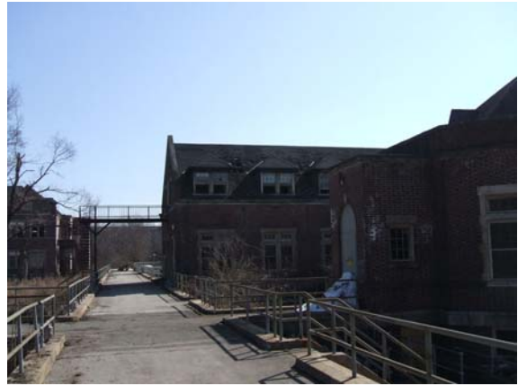
Dietary Building/Franklin Hall Roof
