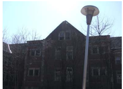
Devon Hall North Parapet
