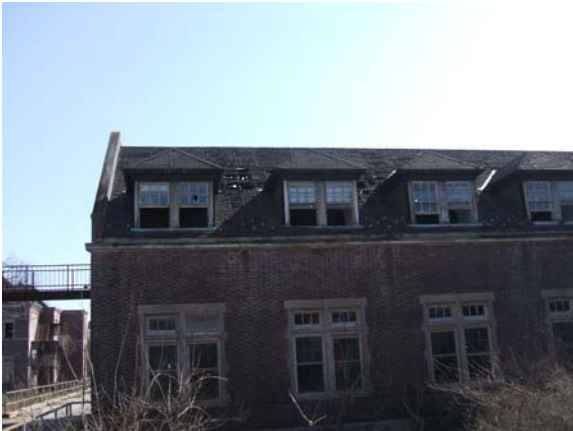
Dietary Building/Franklin Hall Roof
