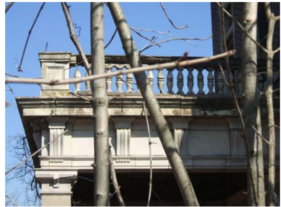
Administration Building Side Porch
