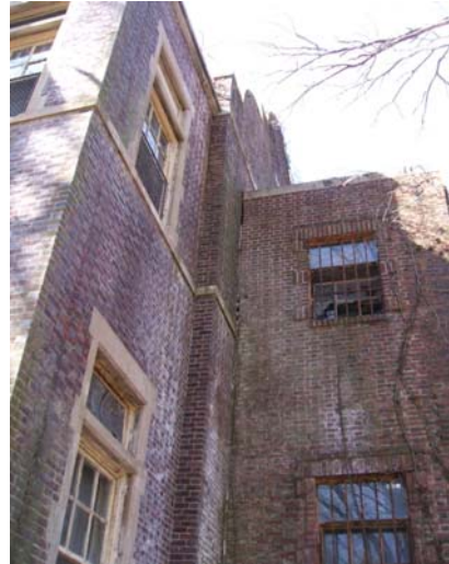
Tincum Hall Stair Tower
