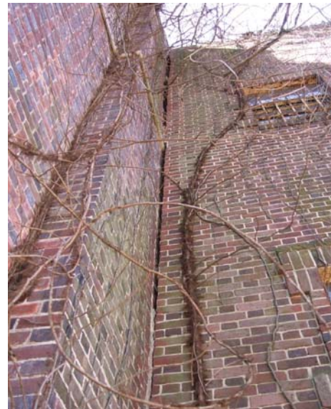
Mayflower Hall Stair Tower
