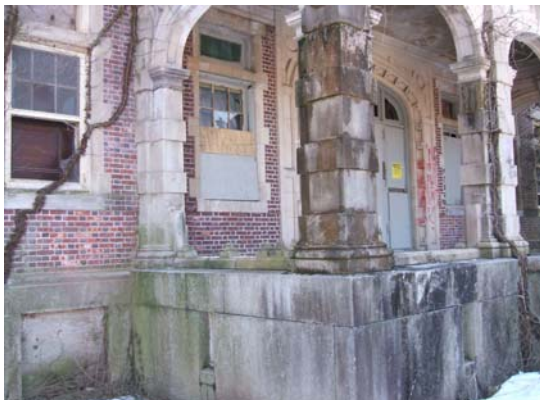
Administration Building Front Porch
