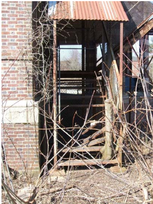
Industry Hall Fire Escape
